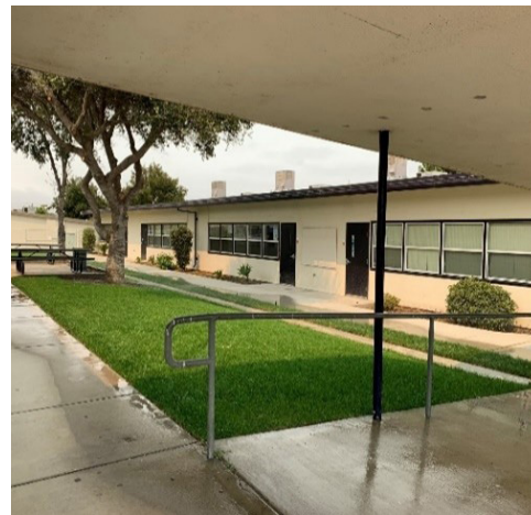
Orcutt Academy High School Restroom Modernization
