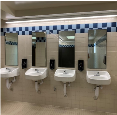
Orcutt Academy High School Restroom Modernization
