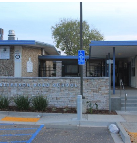
Patterson Road Elementary School Site Safety & Security
