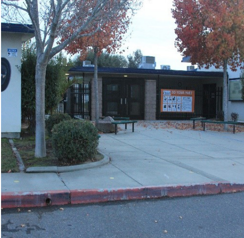
Orcutt Academy High School Site Safety & Security
